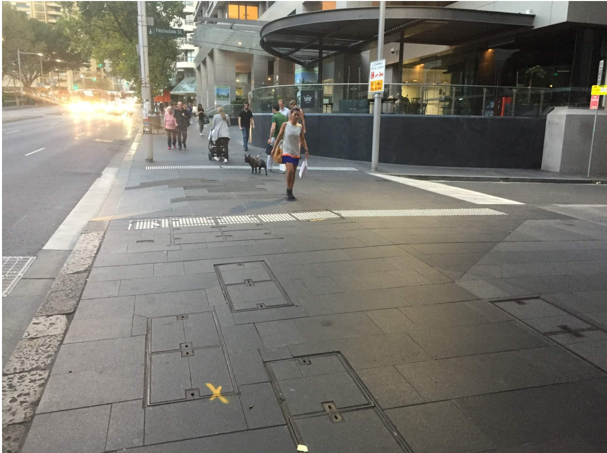
Figure 23 Raised threshold example - cnr Nithsdale and Liverpool Streets
